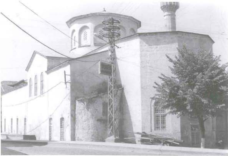
4 The Panagia Chrysokephalos from the south-east. The main pentagonal apse dominates the eastern façade, and the small south apse is a later addition
